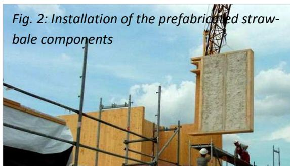
*Fig. 2: Installation of the prefabricated straw-bale components*
